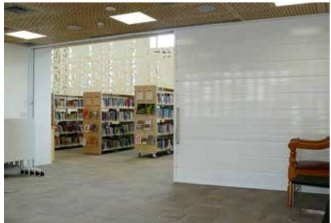
↑ 10 - White powder coated CS AluMax used to screen off an area in a library when required.
