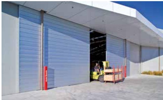
↑ 7 - A natural anodised CS AluMax as an external Bi-Parting surface sliding factory door.
