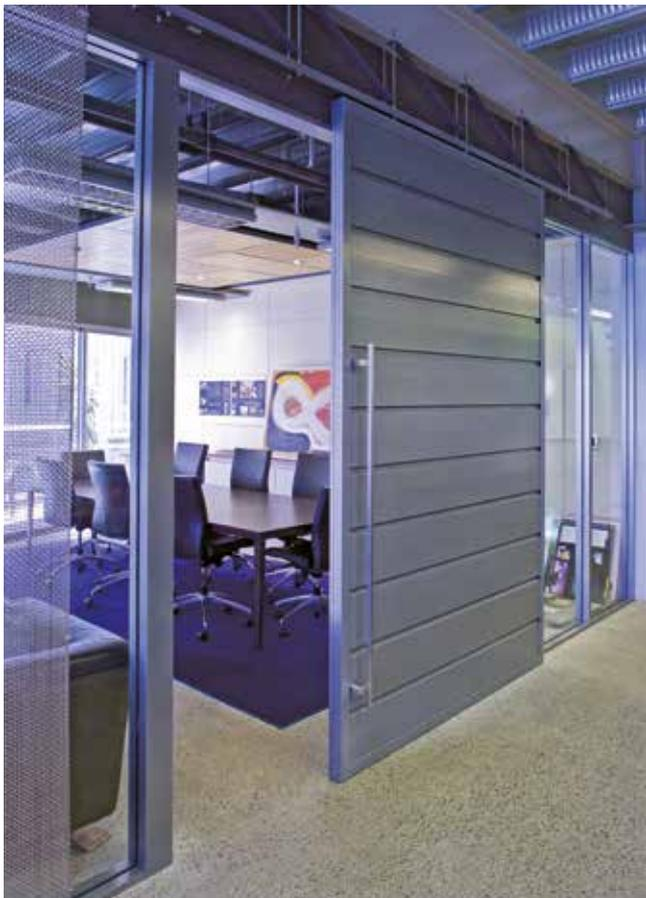
↑ 5 - A powder coated CS AluMax hung from CS HeavyDutyTrack.
