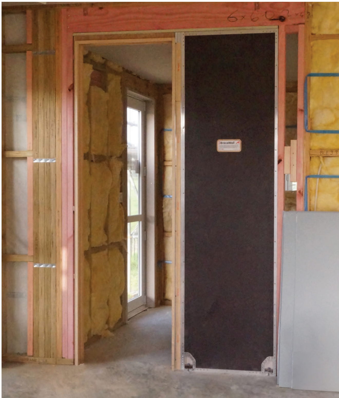
CS BraceWall unit installed into timber framing
